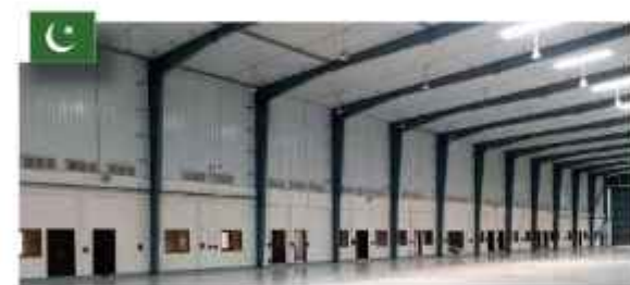
Air Force hangar Pakistan | HANGAR
